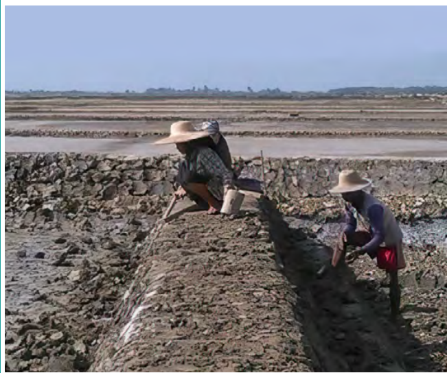
PLATE 21 Manual compacting of dykes
